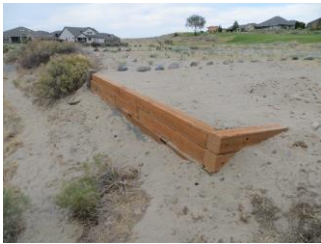
Retaining wall constructed next to the new Grayhawk planting area.
