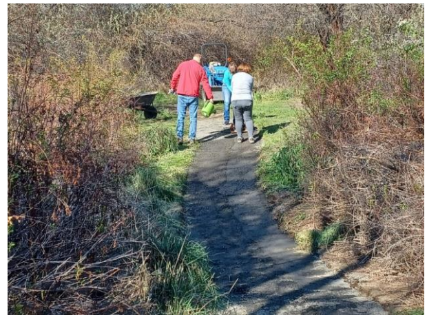
Compacting the final gravel layer
