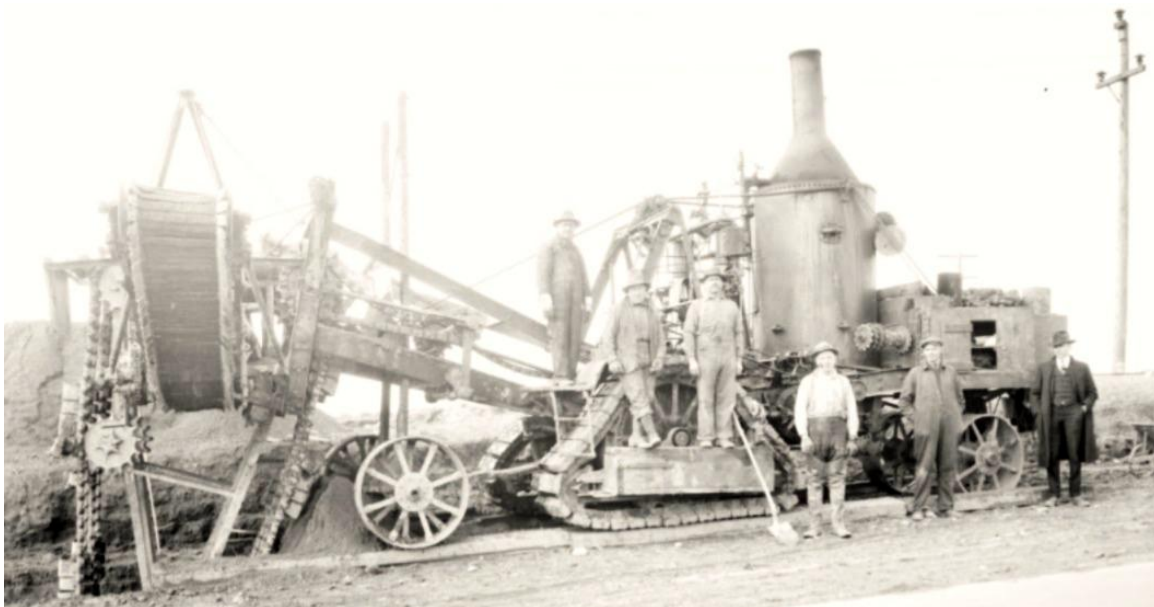
A ditch digger machine for a local canal
