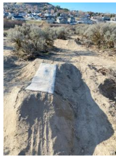
Bicyclist damage in ACNP
